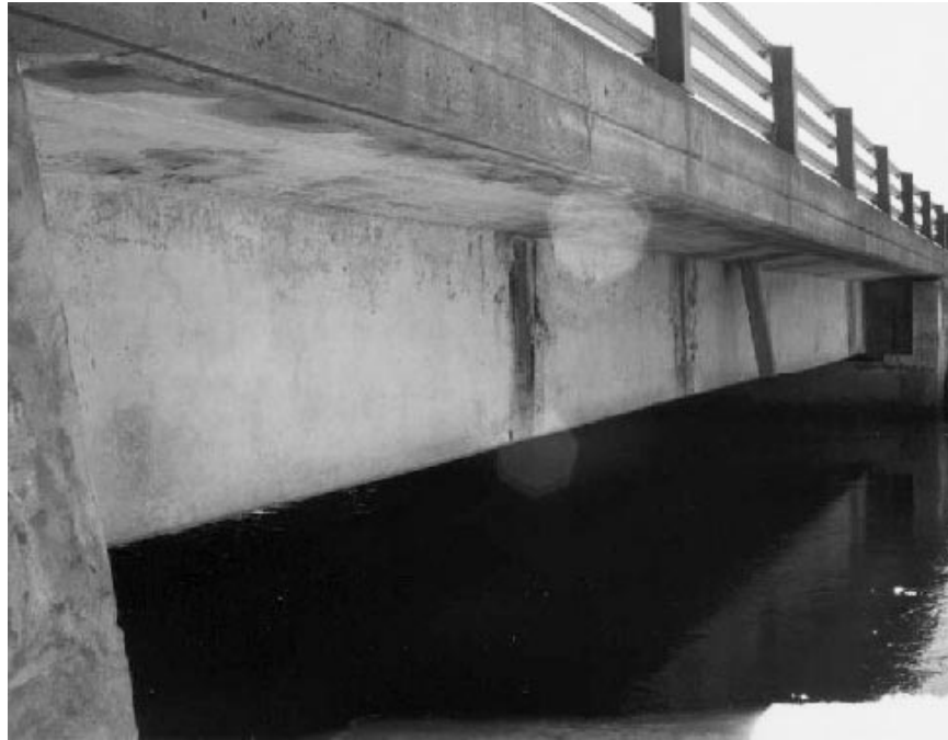
Fig. 1. View of the Sainte-Émélie bridge.
